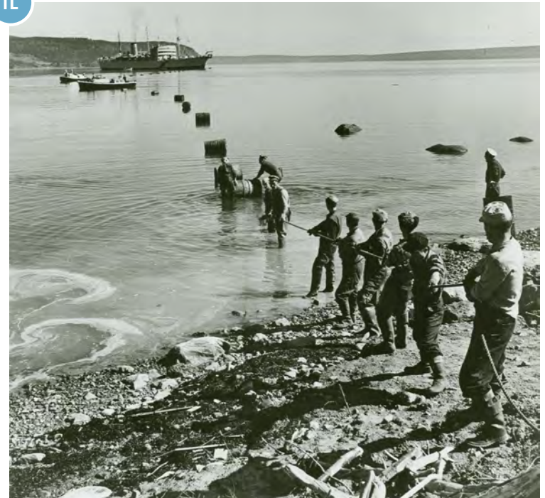
AT&T, Transatlantic Telephone Cable (TAT-1) Pulled Ashore at Clarenville, Newfoundland, ca. 1955. Reproduction Courtesy of the AT&T Archives and History Center.
